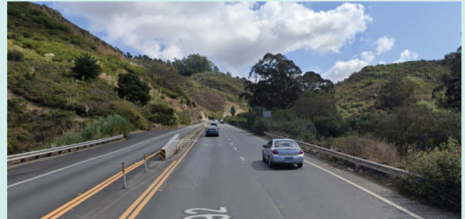
Google Street View of Highway 92 existing passing lane
