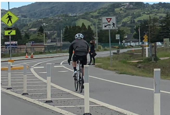
Example of bike lane with flex posts
