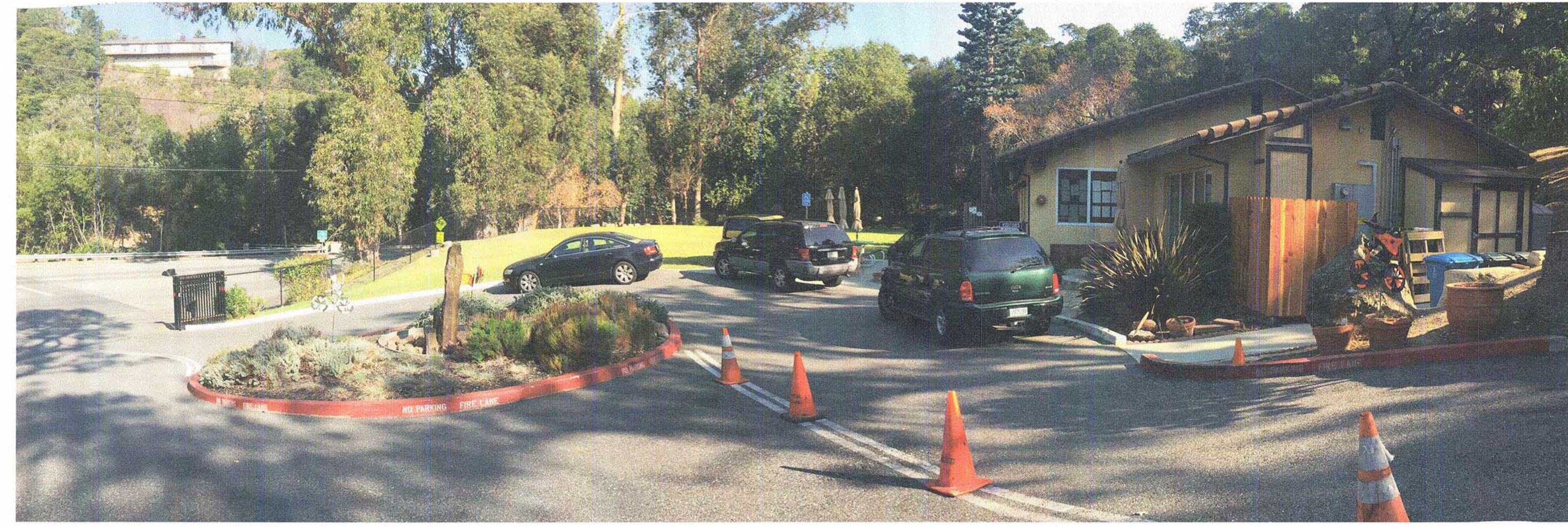
EXISTING SITE PHOTO - MAIN ENTRY • EXISTING BUILDING 'A' 3
