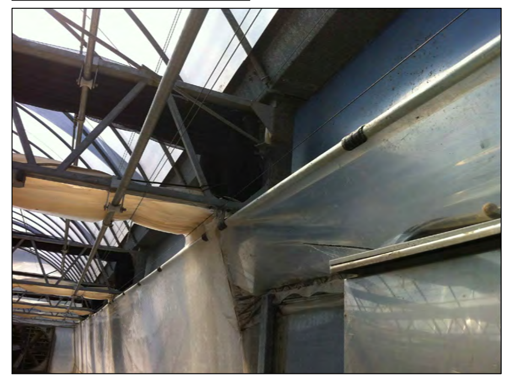
WALL X-BRACE CONNECTION
