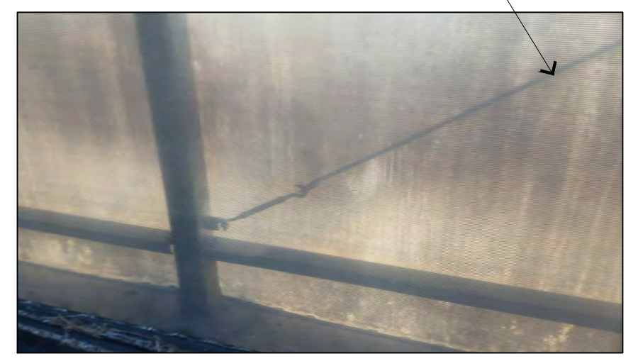
WALL X-BRACE CONNECTION
