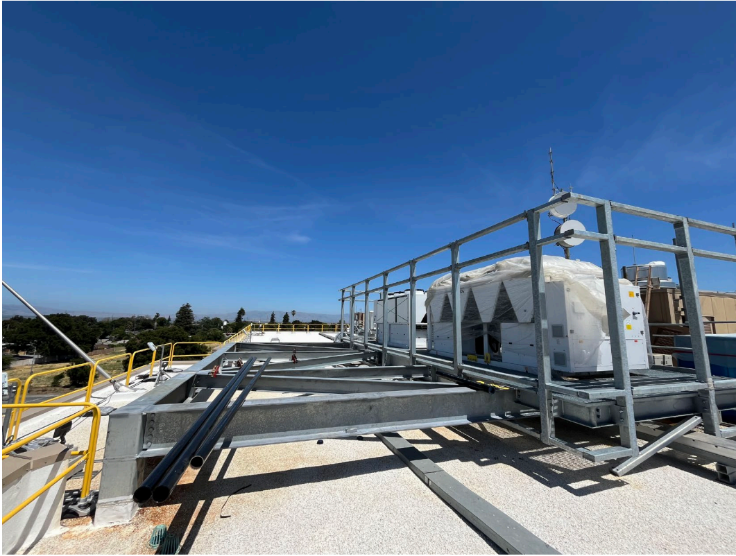
New rooftop mechanical systems installation creating an all-electric building
