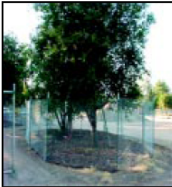
IMAGE 2.15-1 Tree Protection Fence at the Dripline
